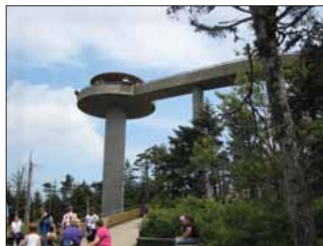
Figure 23. Clingmans Dome observation tower.
