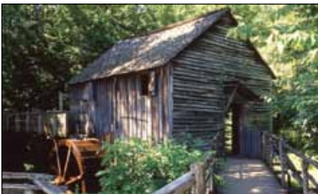
Figure 4. John Cable Grist Mill with flume and wooden water-powered wheel with 40-wheel-buckets on left side of mill and wooden walk-way to entrance.
